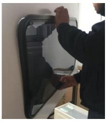
1.2 Step 2: Please apply polyurethane sealant on the outside of the rubber strips and evenly to the border of the frame. The purpose of the strips is only to reduce the amount of glue applied and they cannot replace sealants.
