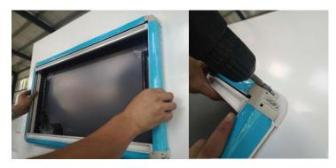
1.5 Step 5. Please attach the 4 cover to the blind along the card slot and mark "L" or "R" on the inside of cover . Finally, tear off the protective film .
