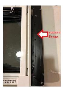
Step 6: The blind is aligned with the installation hole, evenly distance from top to bottom to side of installation hole, there is groove between the inner edge of blind with window to match up the installation. Note: the darkening blind on the lower side, mosquito screen on the upper side.
