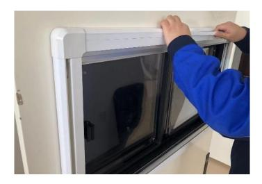
Step 10: Finally, remove the protective flm and the plug of the water hole at the bottom of the window.
