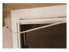
**05** Pull the two ends of the white ribbon to remove the PVC plastic trim from the blinds frame, revealing the installation groove.
