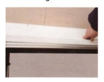
**07** After installation, clip the PVC strip back in to conceal the screws.
