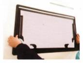
**03** The window is aligned with the installation hole and then pushed flat against the installation hole. Another person should push against from the outside until all the screws are fixed.
