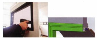
To install the window to the vehicle, use cross groove pan head self-tapping screws provided via the installation clips from the inside. Tighten all screws.
