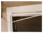
Pull the two ends of the white ribbon to take out the PVC strip from the plastic frame.
