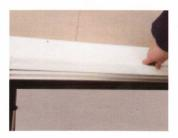
After the installation. Cover up the installation groove back by the PVC strip.
